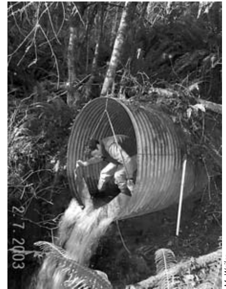
M. Weiler installing v-notch weir in culvert.
